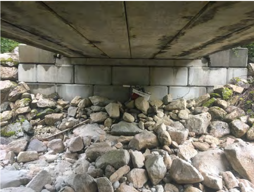
Right Bank Abutment when facing downstream
