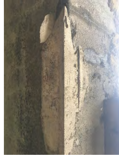
Previous concrete repair
