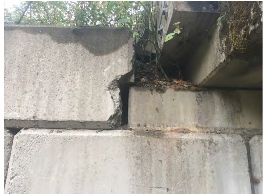
Lock blocks had to shaped around concrete cap at all corners
