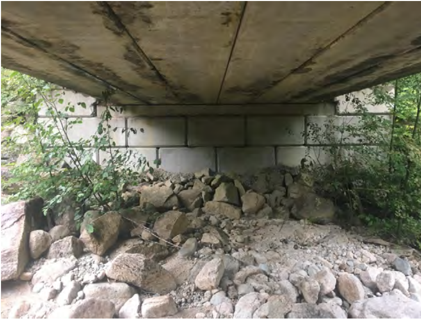
Left Bank Abutment when facing downstream
